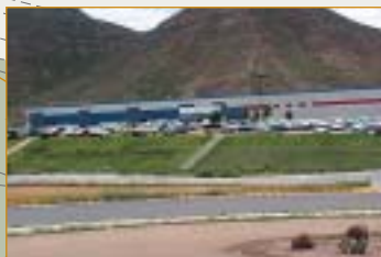
Technotrim, Inc., Saltillo Plant
