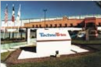
Technotrim, Inc., Ramos Plant
