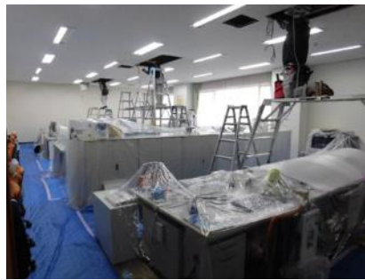
Introduction of energy-saving air-conditioning equipment
