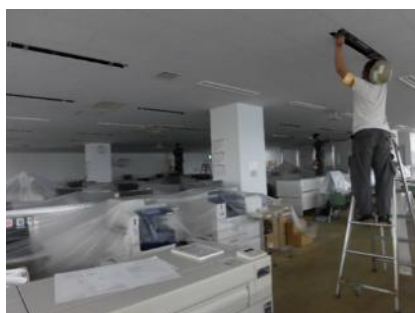
Conversion to LED lighting
